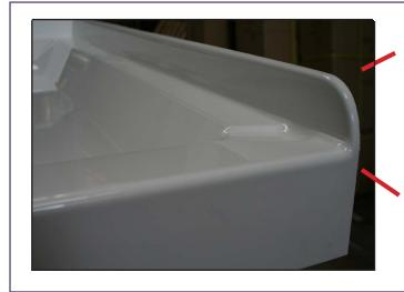
Here is the 40mm high Upstand which is installed hard against the timber framework of the wall. The GIB Board installs down to the top of this, and the Liner is installed over the Upstand and sealed to prevent water entering the walls
